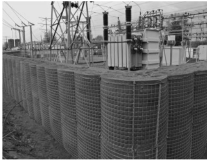
Flood Barrier Source: Con Edison
