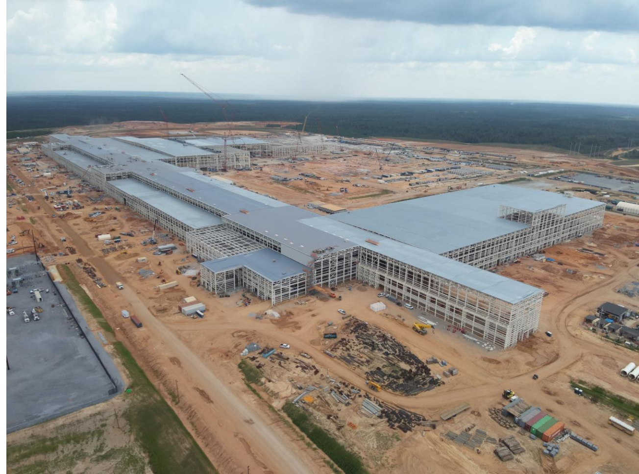
Aerial site view of Bay Minette, July 2025
