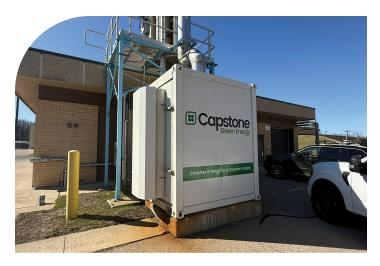
A Capstone microturbine system at the Janesville Wastewater Treatment Plant converts biogas from anaerobic digestion into on-site electricity and heat, boosting energy efficiency and sustainability. The installation includes four C65 and one C200 microturbine, delivering 460 kW of clean, low-maintenance power.
