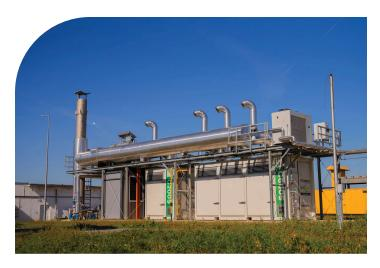
The Capstone C600S microturbine, fueled by biogas, and the C200S microturbine, powered by natural gas, provide a high-efficiency cogeneration solution for the Cristesti Wastewater Treatment Plant. Generating 800kW of clean power while capturing waste heat for sludge drying and heating, the system cuts costs, reduces emissions, and enhances energy independence.
