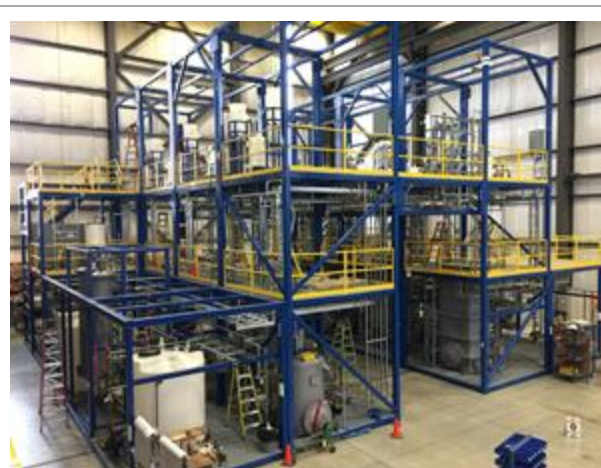
Phase 1 & 2 Modules – photograph taken May 29th, 2019
