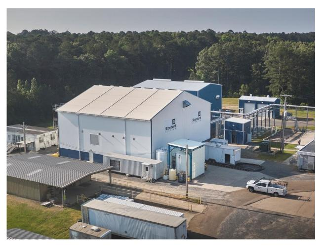
In May 2020, the Company commissioned its industrial-scale DLE Demonstration Plant at LANXESS' South Plant. The Demonstration Plant, which is the first-of-its-kind in the world, utilizes, among other technologies, the Company's proprietary DLE process to extract lithium from LANXESS' post bromine extraction tail-brine.
