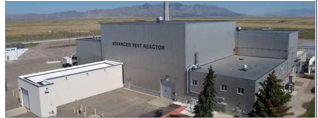
INL's Advanced Test Reactor (ATR)
