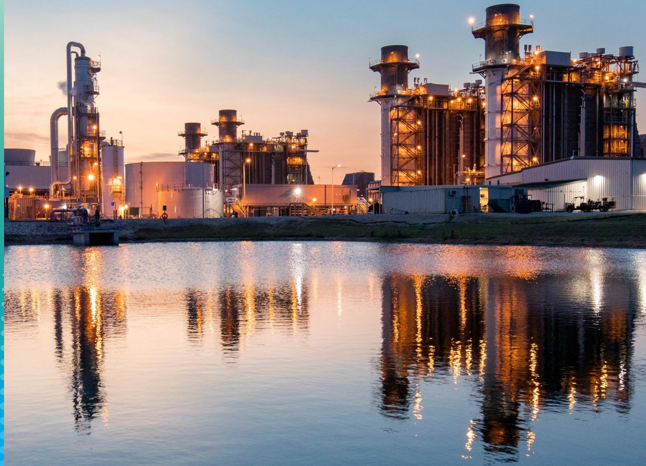
Temple Power Plants Bell County, Texas
