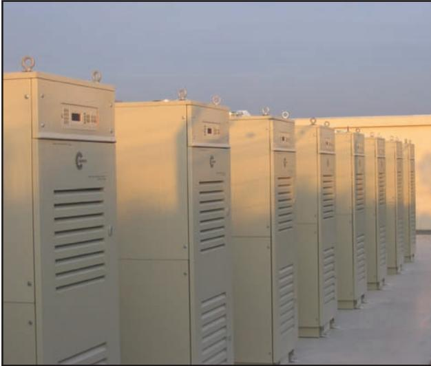
**Each of the 18 Capstone microturbines in La Ciotat is rated 65 kW. Maintenance is simplified, Verdesis said, by the fact that each microturbine unit has just one moving part.**
