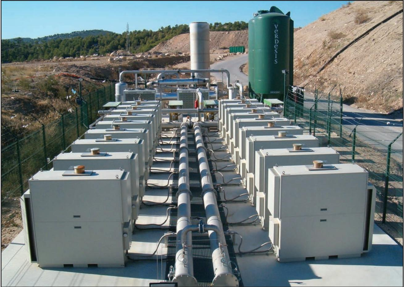
In a project that has turned waste into energy, Verdesis, the Capstone Turbine distributor for Belgium and France, has installed 18 microturbines in La Ciotat, France. The microturbines use waste gas from decomposition to generate 1.2 MW of electricity — enough to power 2000 homes.
