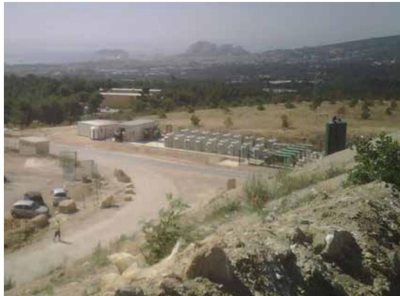
*Eighteen C65 microturbines running on methane gas generate power and heat at La Ciotat Landfill in France.*
