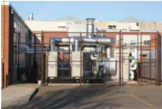
A PureComfort® trigeneration solution featuring four 65kW Capstone microturbines provide cooling, heating, and onsite power for Branford High School in Connecticut.
