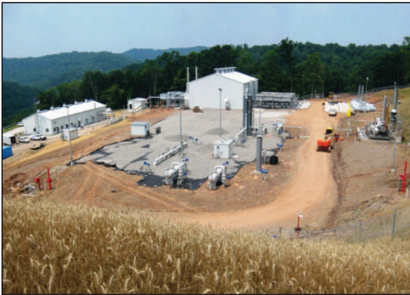
Electric power was not economically available at this greenfield natural gas storage facility in West Virginia, U.S.A. Basic Systems Inc.'s design included four Caterpillar G3608/Ariel JGC/6 compressor packages. Nine Capstone model C65 microturbines provide all the power for the site.
