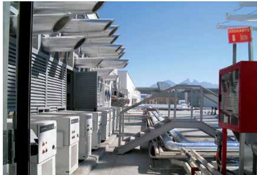
*Twenty Capstone C65 microturbines produce 40 percent of the electrical power needed to operate a department store in Monterrey, Mexico.*
