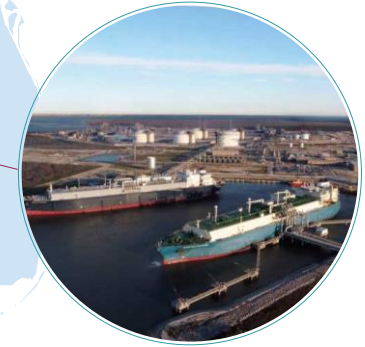
Sabine Pass Liquefaction ~30 mtpa Total Production Capacity
