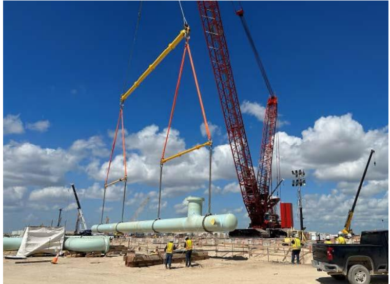
Underground Feed Gas Fabrication
