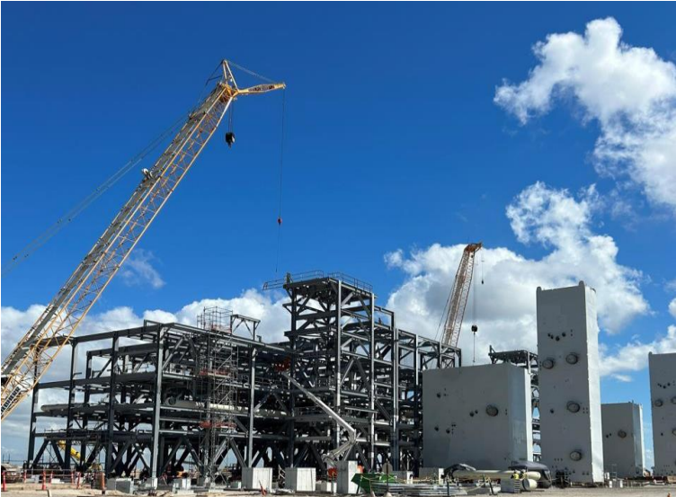
Train 1 Cryo Rack Structural Steel Installation
