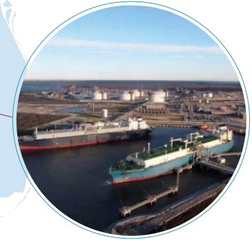
Sabine Pass Liquefaction ~30 mtpa Total Production Capacity
