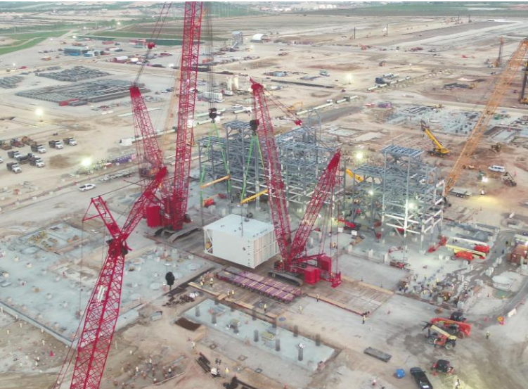
Train 1 Cold Box Installation
