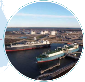
Sabine Pass Liquefaction ~30 mtpa Total Production Capacity
