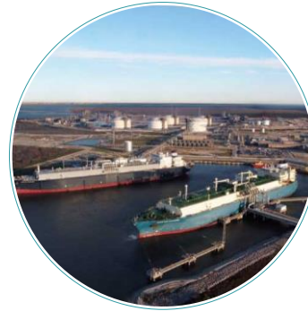
Sabine Pass Liquefaction ~30 mtpa Total Production Capacity
