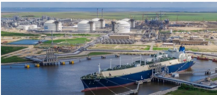
Sabine Pass Liquefaction Project
