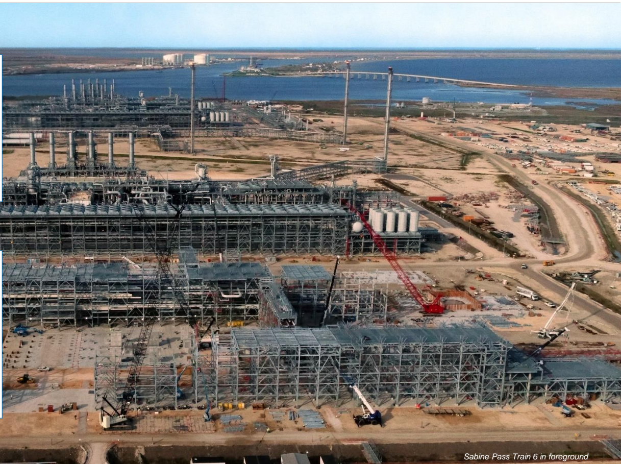
Sabine Pass Train 6 in foreground
