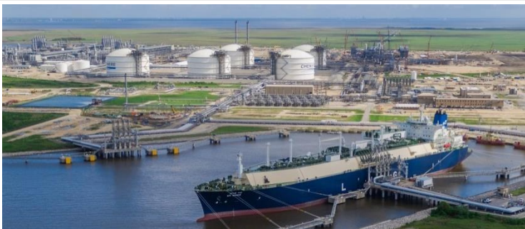
Sabine Pass Liquefaction Project
