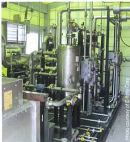
The gas conditioning skid at the York, Pennsylvania WWTP removes moisture, hydrogen sulfide and siloxanes from the biogas.
