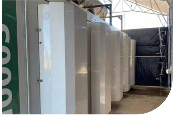
**One C1000S Microturbine fueled by liquid natural gas provides the Ascend Growing and Processing Facility in Denver, Colorado with electricity, heating, and cooling while reducing the facility's carbon footprint.**
