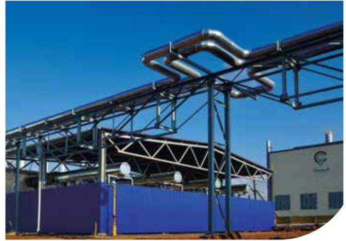
Four natural gas fired Capstone C1000 microturbines operating in a CHP application produce 4MW of clean and reliable power as well as 4.8MW of thermal energy for the Slutsk Cheese Factory.
