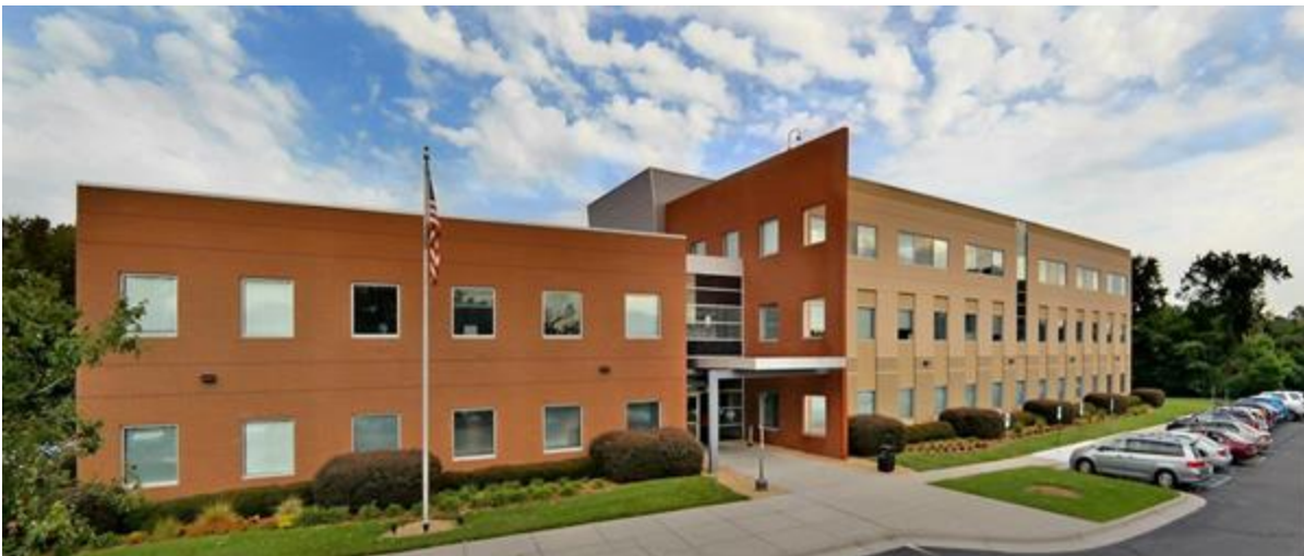
Social Security Administration Building, Norfolk, Virginia
