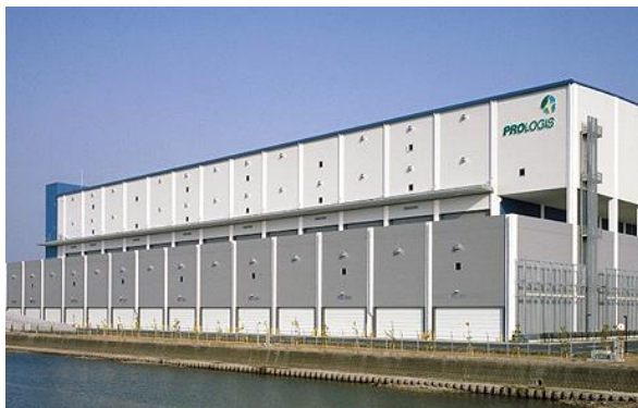
Prologis Park Yokohama Tsurumi, Japan
