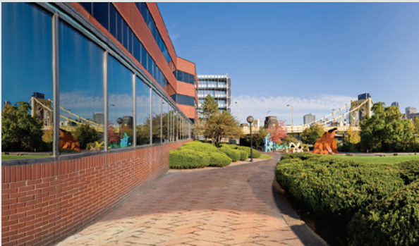
On the cover: Matthews International Corporation's corporate headquarters, located on the NorthShore riverfront in Pittsburgh, Pennsylvania, USA.
