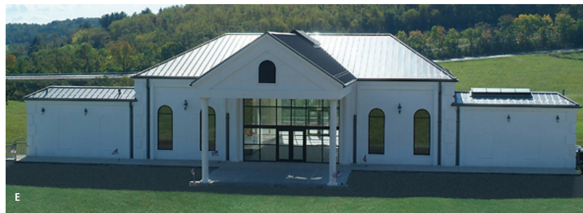
(E) Community Chapel Mausoleum – A two-story mausoleum was constructed by Matthews' Gibraltar Mausoleum Construction Company for Woodruff Memorial Park in Canonsburg, PA. The mausoleum includes over 1000 interior and exterior crypts and a library of 700 niches.
