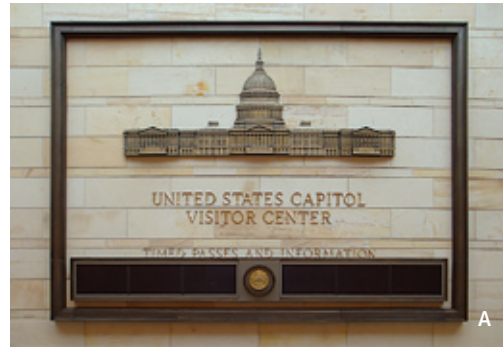
(A) Capitol Visitor Center Signage – Two 15-foot-long x 7-foot-high sculpted, aluminum castings of the Capitol Building with identifying letters were manufactured for the United States Capitol Building's new visitor center in Washington, D.C.
