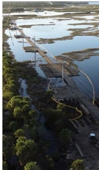
Kinbro temporary roadway.
