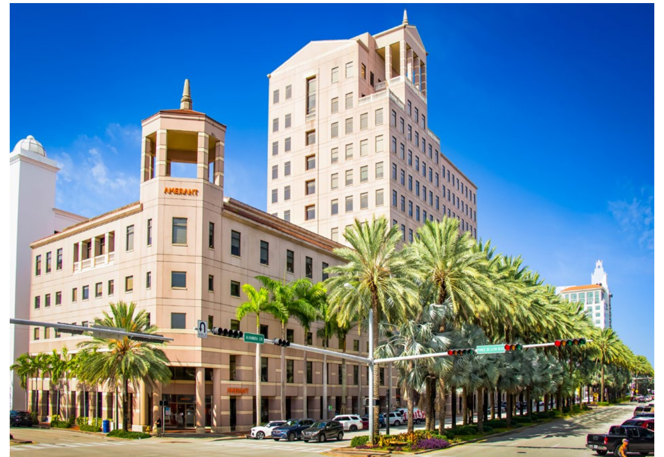
Amerant Bank Headquarters in Coral Gables, Florida.
