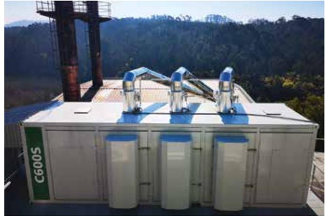
*To support an increase in production capacity, plant officials sought an efficient solution for their plant expansion. Rather than import more power from the local utility at extremely high rates officials installed on-site microturbine CHP solution.*
