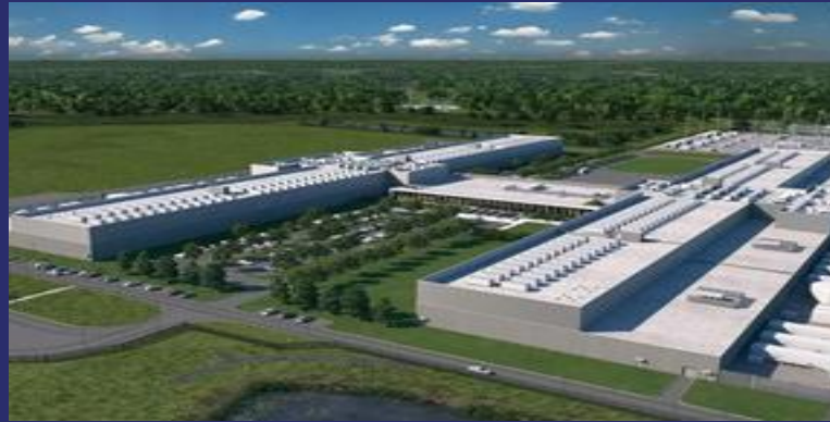
QTS Data Centers NOVA & Metro Richmond, Virginia
