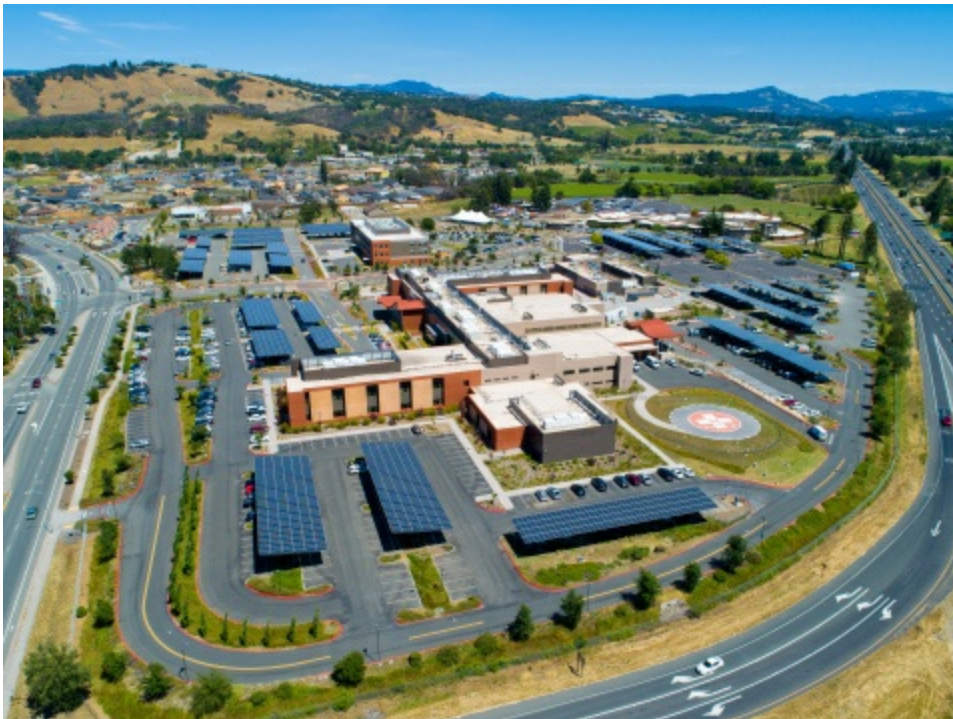
Sutter Santa Rosa Regional Hospital's 1.6 megawatt solar energy generation installation (Photo: Business Wire)
