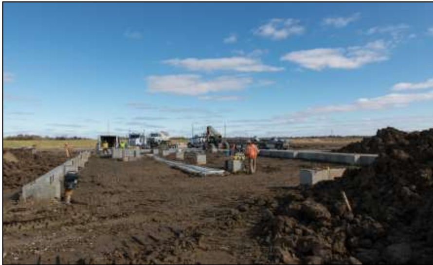
Foundations for the Poplar Grove Mine's CHPP
