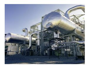
JEFFTREAT® and DGA Agent® gas treating amines help refineries to more effectively capture sulfur from off gases to reduce atmospheric emissions.
