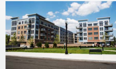
Portside at East Pier
