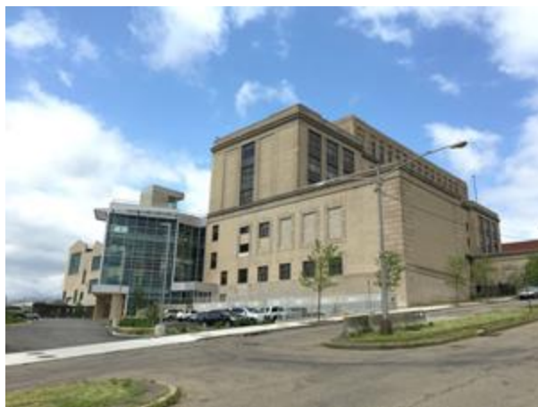
(2) Capstone C65 Microturbines provide Combined Cooling, Heating & Power (CCHP) to the Energy Innovation Center in Pittsburgh, Pennsylvania.
