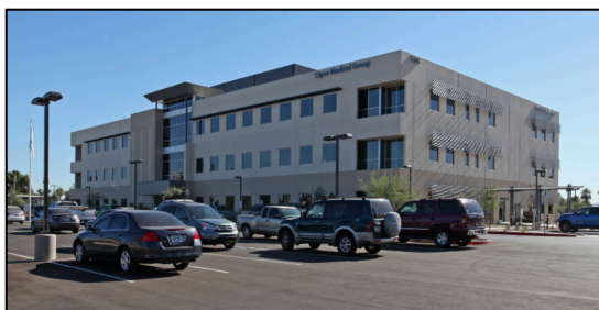
3003 North 3 rd Street, Phoenix, AZ
