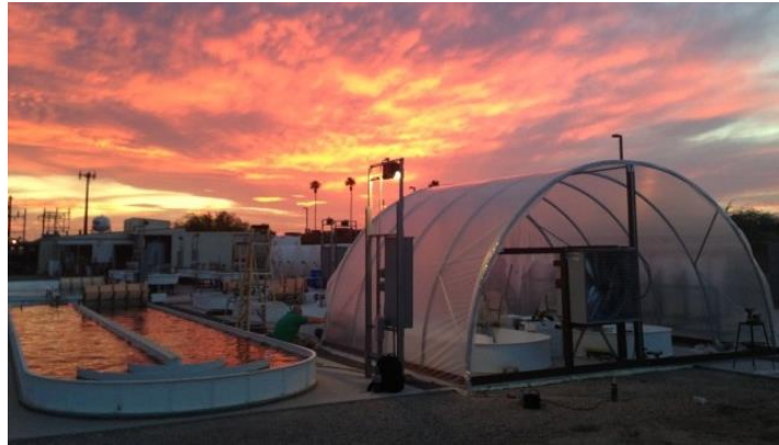
Covered pond at Arizona Center for Algae Technology & Innovation facility
