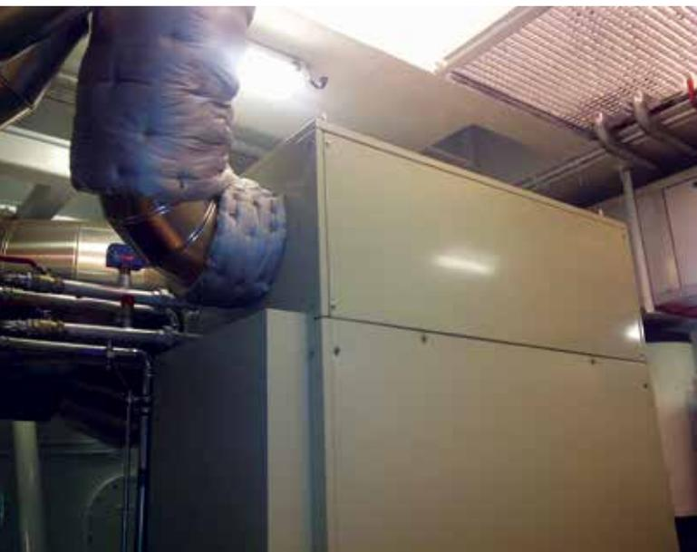
Two liquid natural-gas fueled Capstone C30 MicroTurbines onboard the MTS Argonon Type C tanker in Rotterdam, Netherlands, operate in an N+1 setting and serve as the main electrical power supply.
