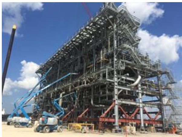
Finishing touches for the secondary transfer-line exchanger module at Gulf Island's fabrication yard in Houma, Louisiana.
