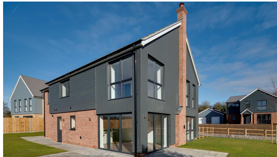
New construction luxury development in Hertfordshire, UK utilizing ColorPlus® HardiePlank® on exteriors
