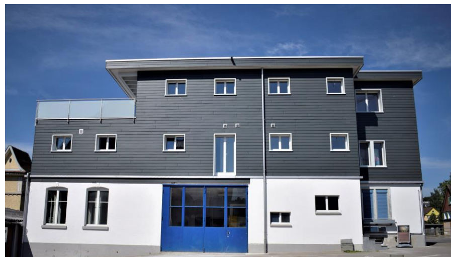
New construction in Eastern Switzerland utilizing ColorPlus® HardiePlank® on the exteriors and Fermacell fiber gypsum interior wall linings
