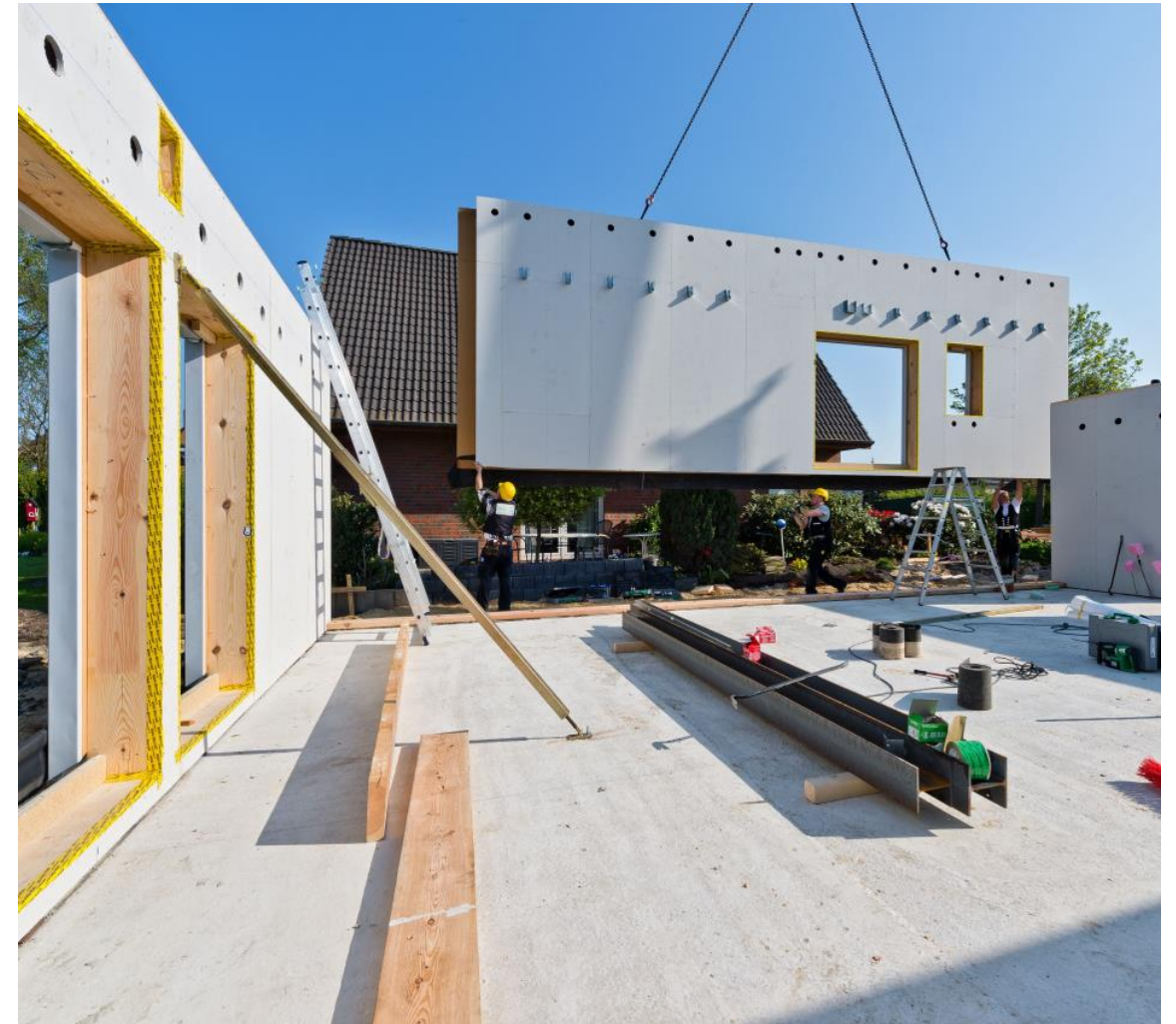
Pre-fabrication construction in Germany
