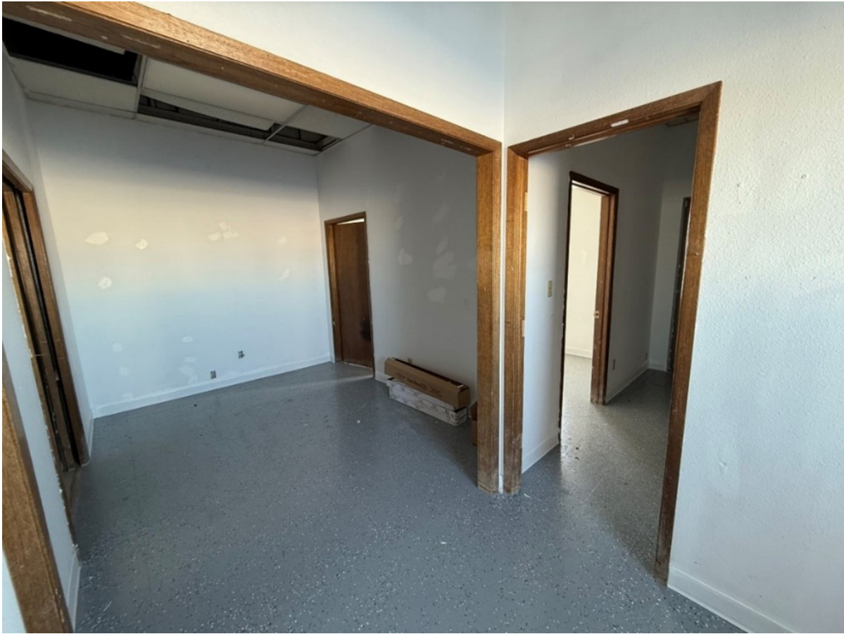
Interior of the conventional mine medical building that is being updated for office and warehouse space. Total square footage of 2,800.
