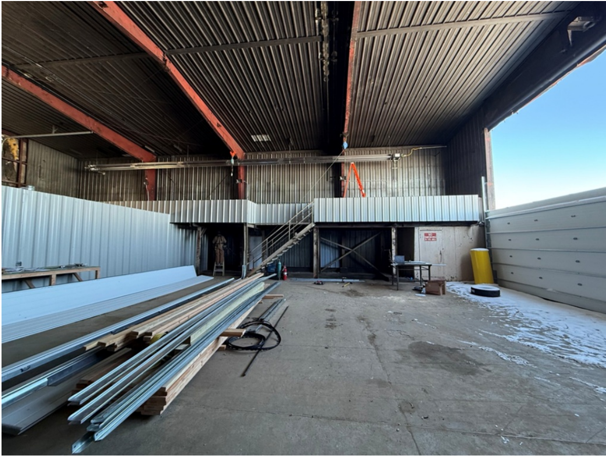
Interior of the conventional mine "wash bay" that is being updated for use as a drilling and logging building. Total square footage is 4,400.
