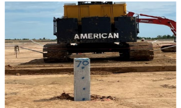
Pile driving underway
