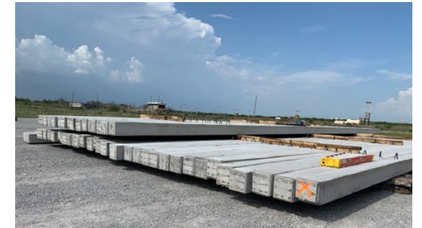
First piles delivered to site
