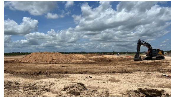
Plant 1 site preparation
