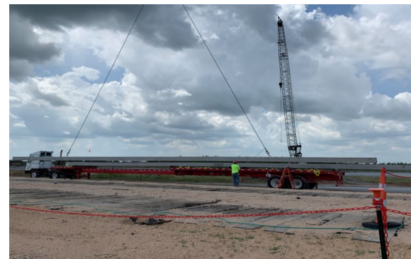
Site prep for piling
